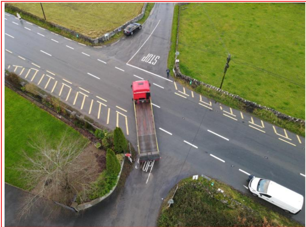
Note that absence of kerb radii determines that HGV turning movement has to cross lane to contraflow lane to turn left.
