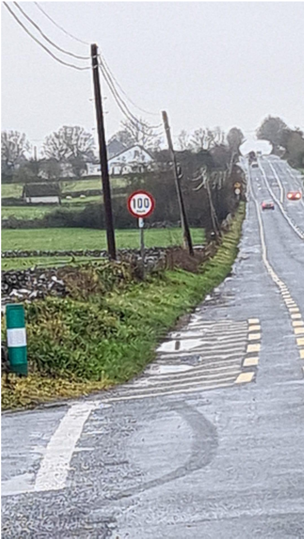
Note this photograph of 26/11/2025 shows Stop line at inside of carriageway edge from L-6146 on Eastern side of N83 facing Galway
